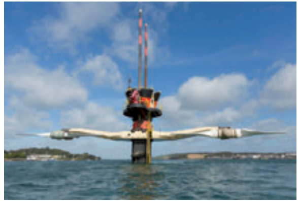
Figure 5.2-5 Ocean-current power plant (SeaGen). The turbines can be raised out of the sea for maintenance purposes. Source: The image was made available by Marine Current Turbines, a subsidiary of Siemens AG
